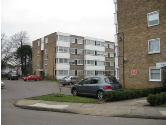
Photograph 5: Black AC infill panels between external windows.
