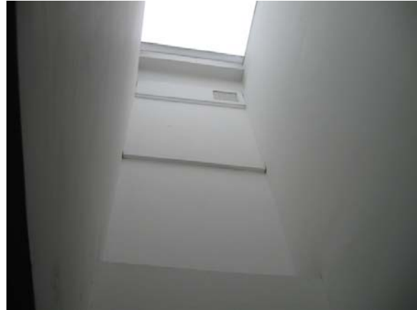
Photograph 2: No access was possible to the Skylight's present in the Corridor on the Second Floor
