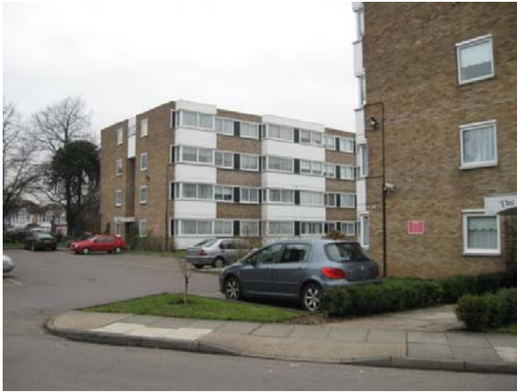
Photograph 5: Black AC infill panels between external windows.
