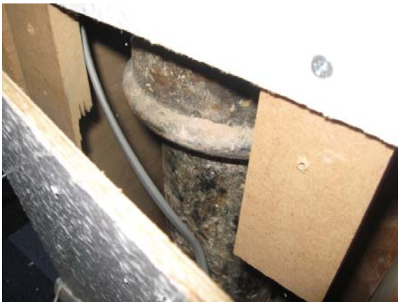
Photograph 3: Example of waste pipe riser identified within the Ground and First Floor Corridors
