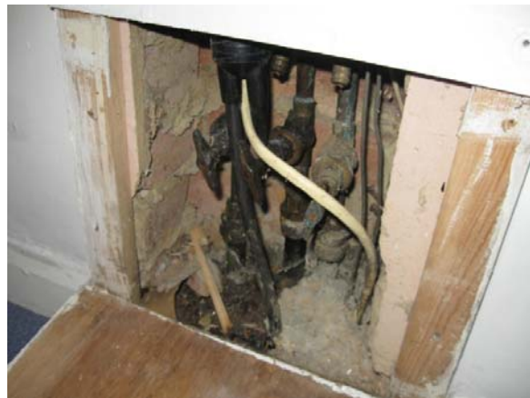
Photograph 4: Example of mains water pipe riser identified within the Ground and First Floor Corridors
