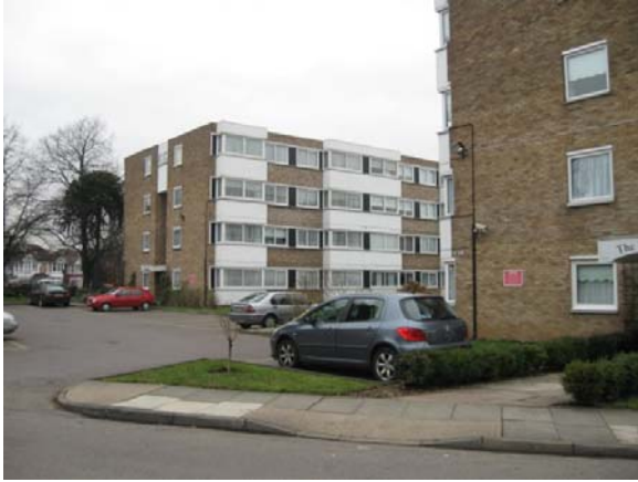
Photograph 5: AC infill panels between external windows.
